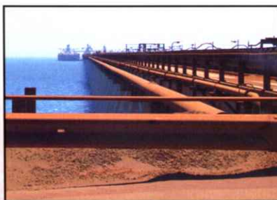
The Ore Wharf at Port Walcott stands 20m above sea level to avoid inundation during cyclonic events. Visiting vessels are laden with diesel fuel and heavy fuel oils.
