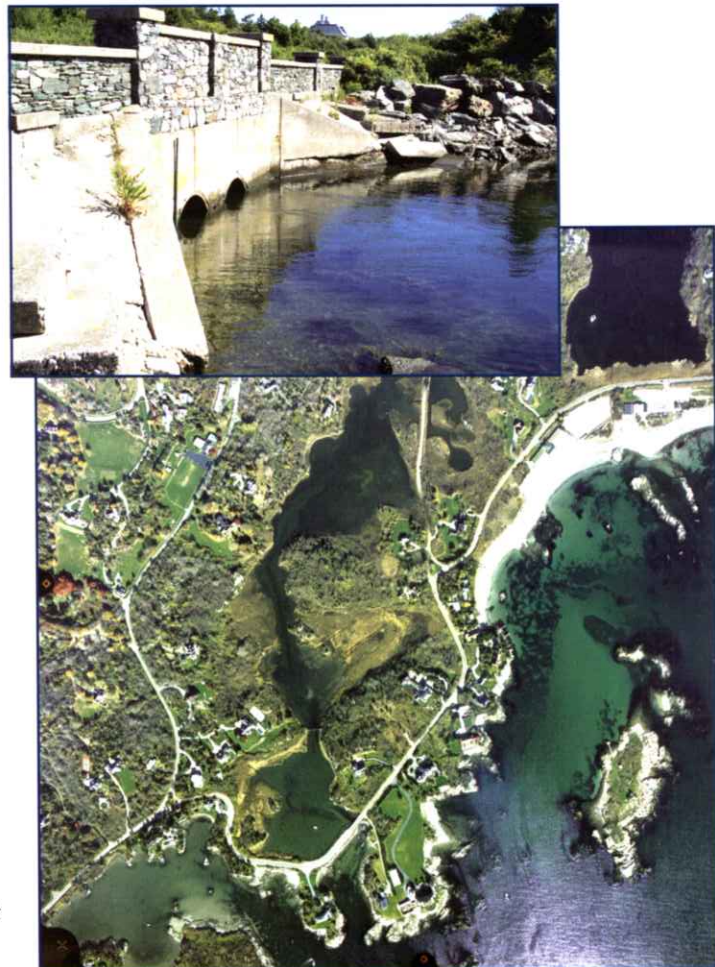
Above photo: A pair of 1.2 m diameter culverts, located beneath Ocean Drive at the mouth of Gooseneck Cove. Aerial photograph courtesy of Save the Bay.
